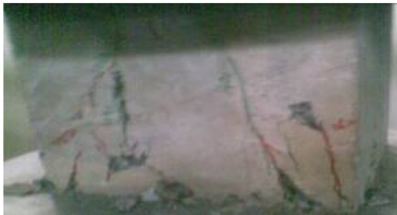
Fig. 7.2 Vertical Cracks leading to Column fragments
